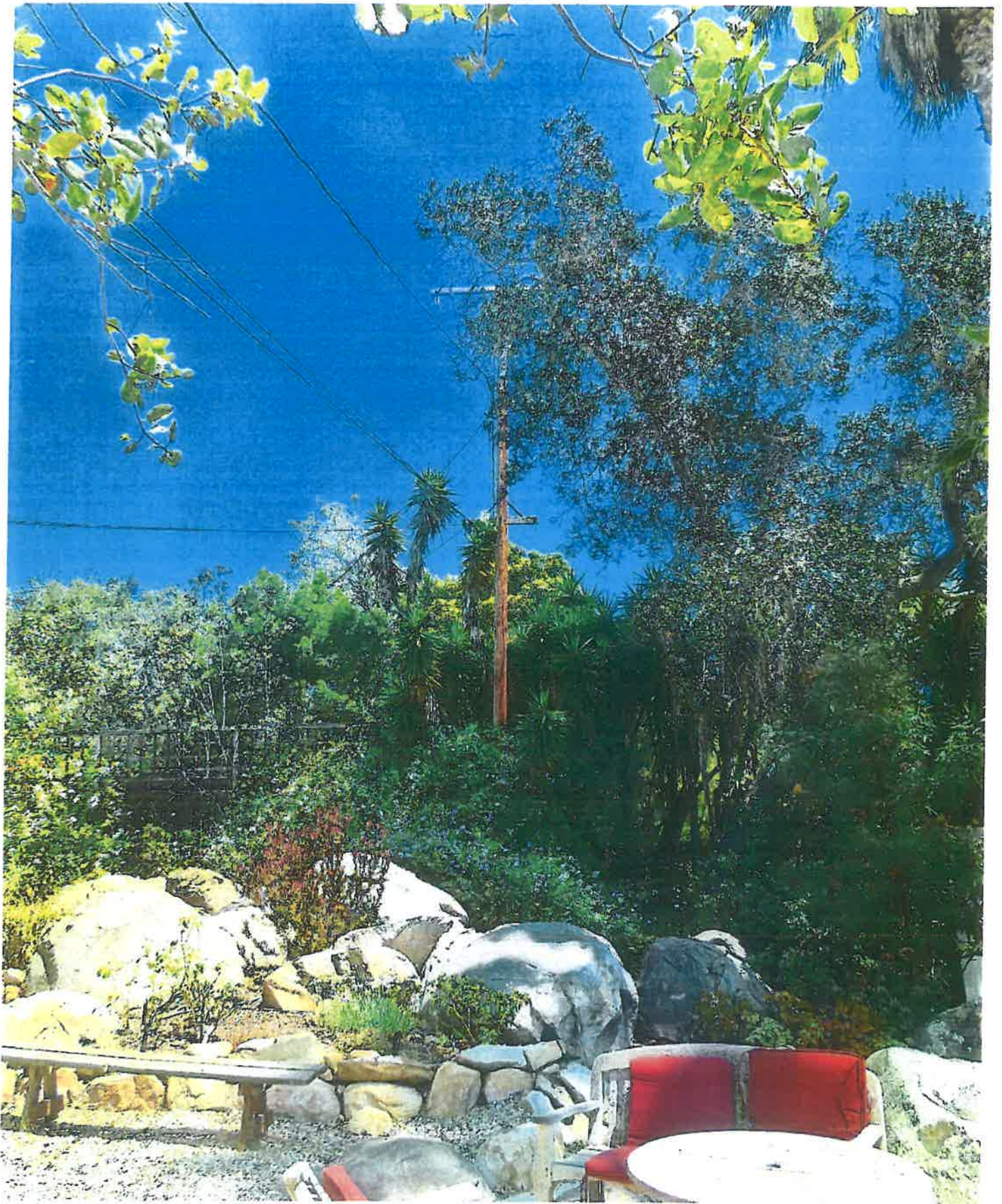
Dist. 49 Deteriorated Pole L / E
