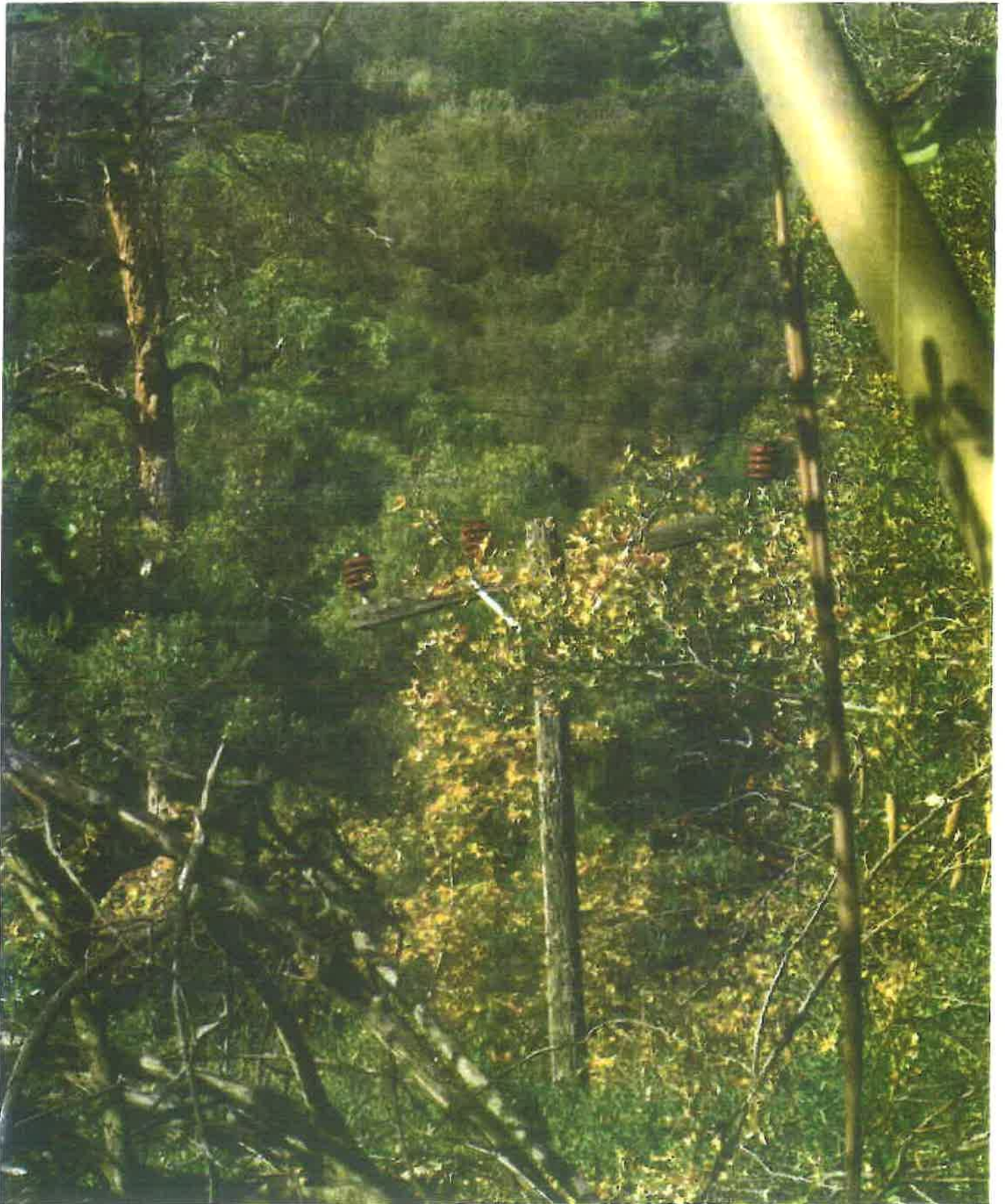
Dist. 49 Deteriorated Pole L / NW
