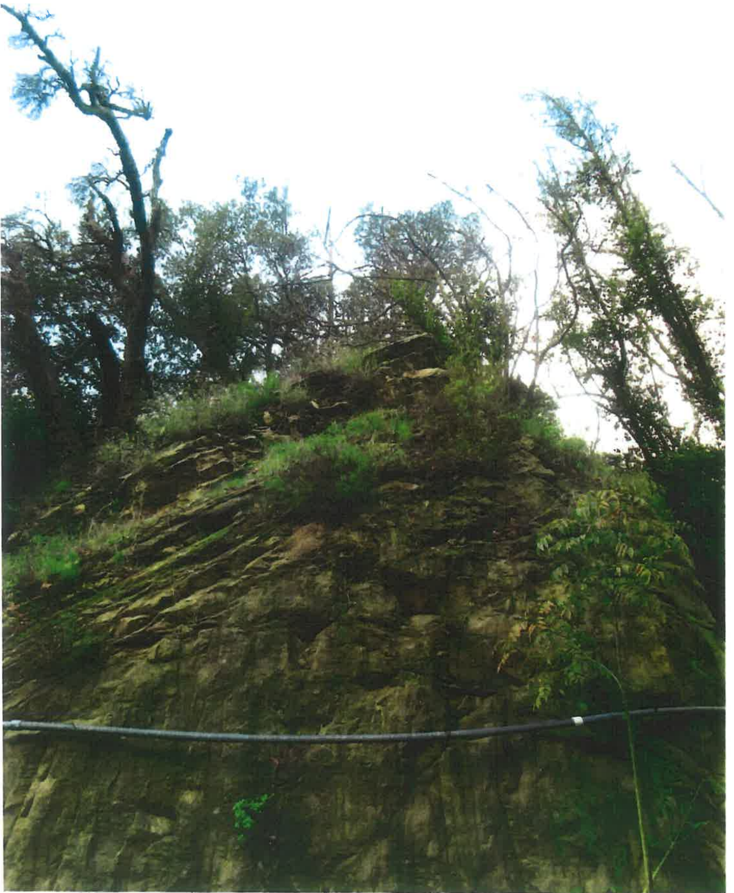
Dist.49 Deteriorated Pole L / W
